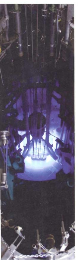
This University of Missouri reactor core could be harnessed to make moly for the short and eventually the long run.
